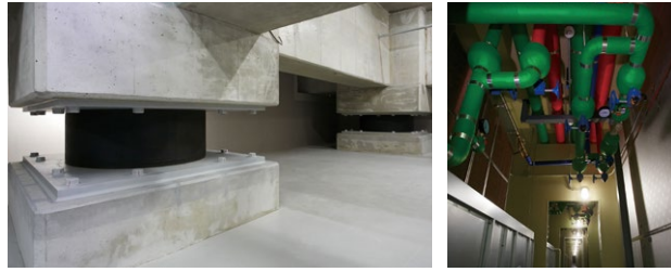
Busan Global Cloud Center : seismic base isolation facility (left) and built-up air conditioning facility
