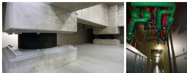
Busan Global Cloud Center: seismic base isolation facility (left) and built-up air conditioning facility
